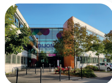
Atrium France services 6, place des Savoirs
